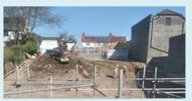
We have had Morgan Sindall on site since January, the demolition of the existing building has taken place, and the site is being excavated at present ready for the foundations and the steel frame to be erected.
